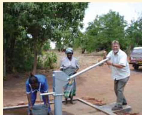
Brian Addy tests out the new pump and well
